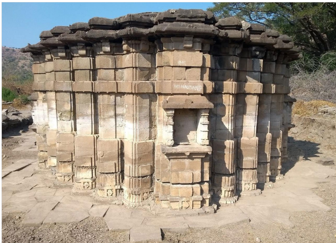
Fig. 3.61: South-facing elevation of the Bagīcā temple
