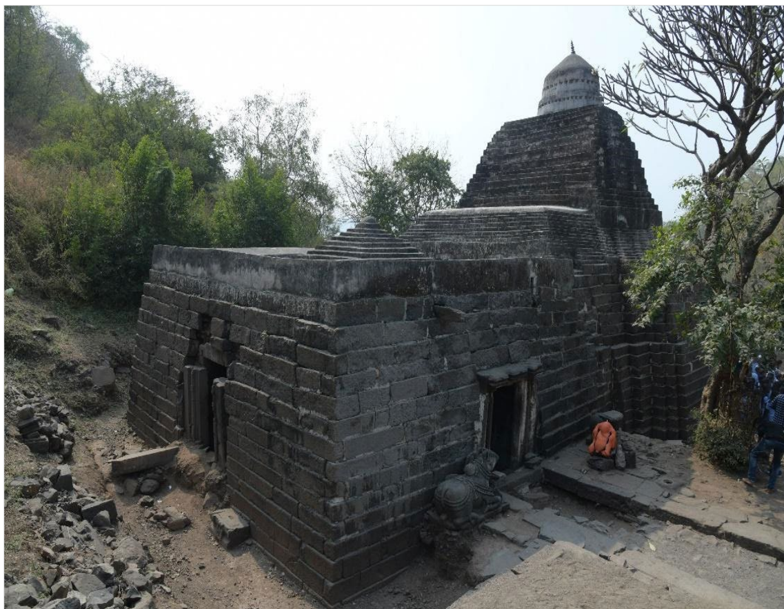
Fig. 3.38: Kumāreśvara temple – View from the north
