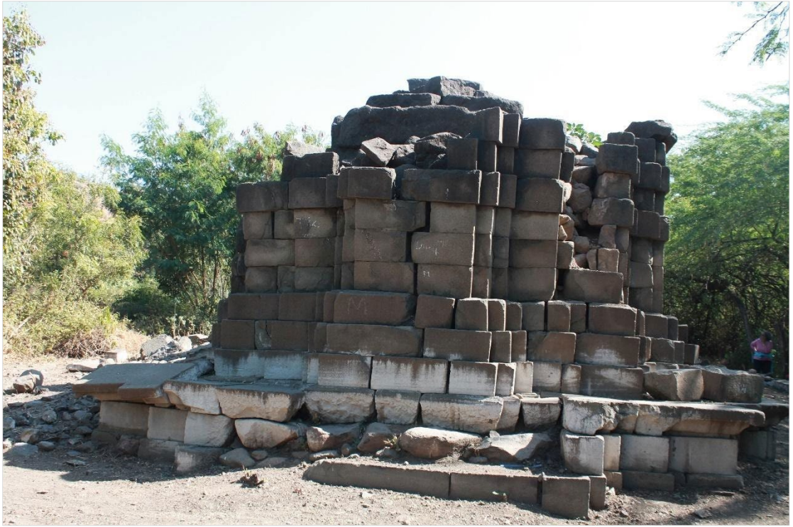
Fig. 3.76: West-elevation of Copadā Temple
