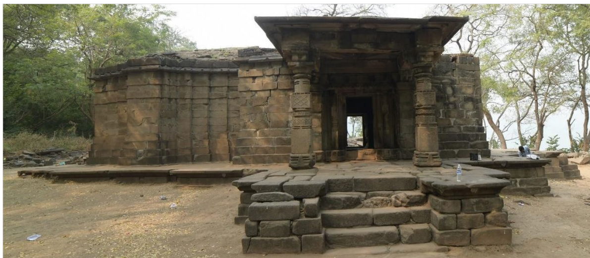
Fig. 3.69: West-facing elevation of Mora temple
