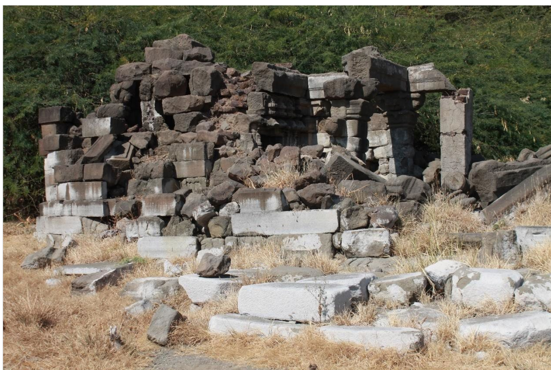
Fig. 3.79: South-elevation of Muṅgalyā temple
