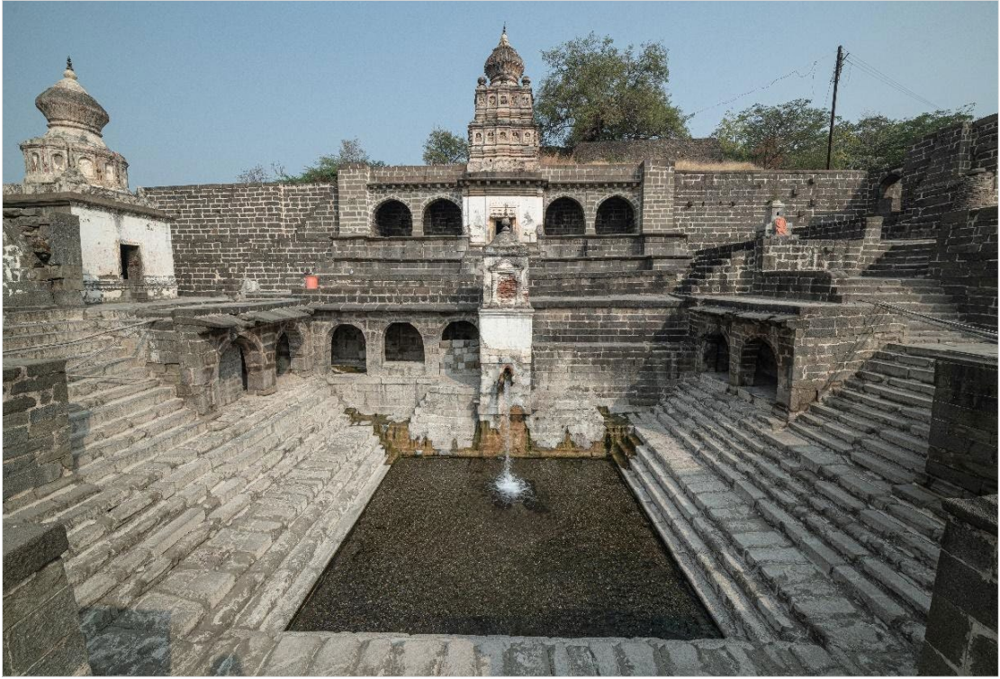
Fig. 3.30: Central Shrine- Viṣṇu temple above the perennial dhāra surrounded by a colonnade
