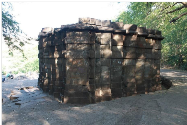
Fig. 3.71: West-facing elevation of Mora temple
