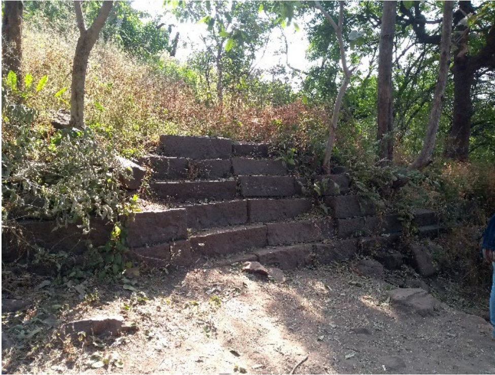
Fig. A.16. Probable remains of prākāra wall before the Yajñeśvara temple.
